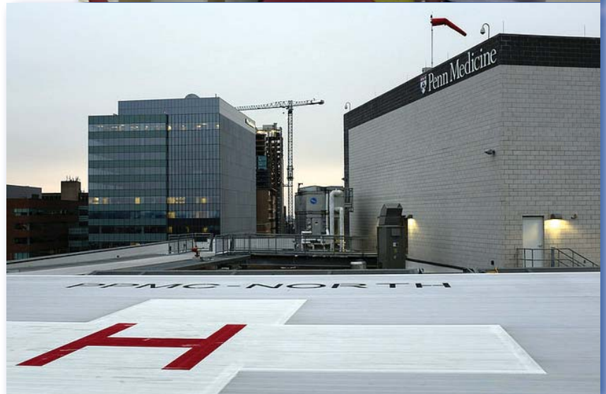
New heavy-duty helipad to accommodate larger helicopters.
